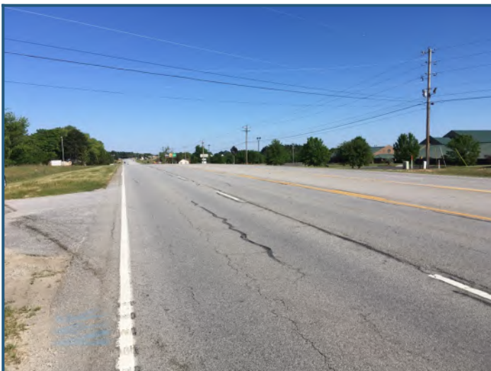
Streetscape: Southeast view of U.S. Highway 378
